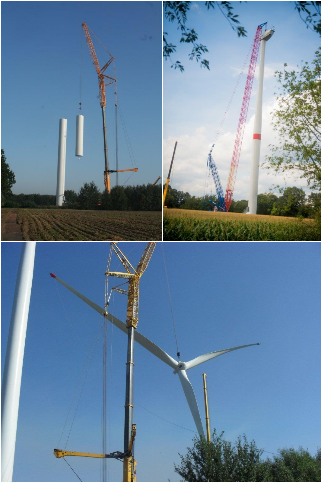
Foto 2: montage windturbines
